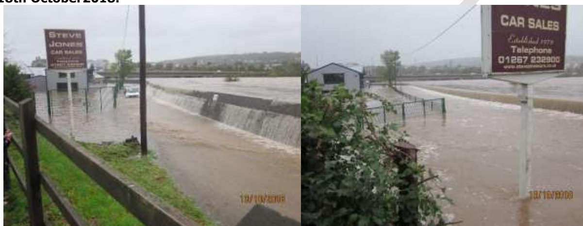
Plate 5 Photographs of the flood defences at Old Llangunnor Road on the afternoon of 18th October 2018.
