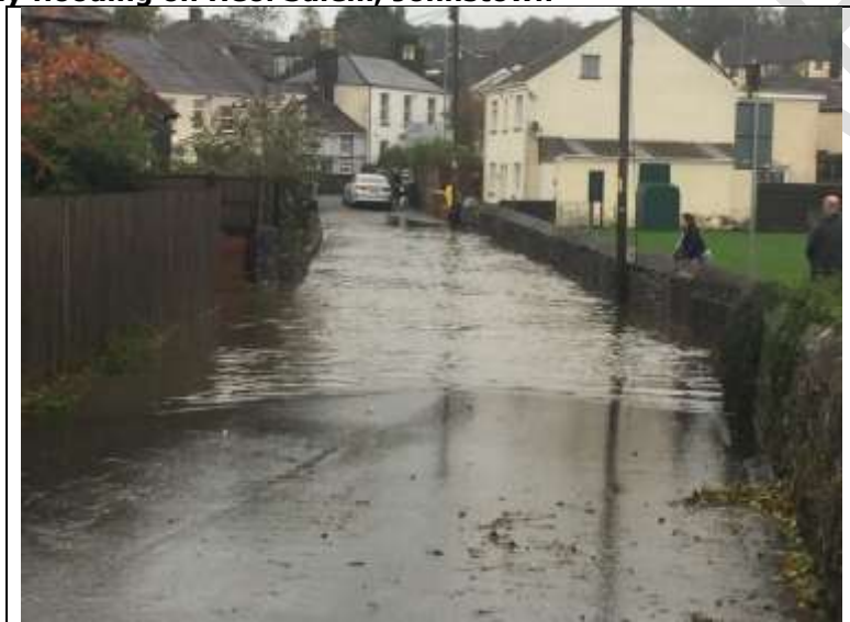
Plate 1: Highway flooding on Heol Salem, Johnstown
