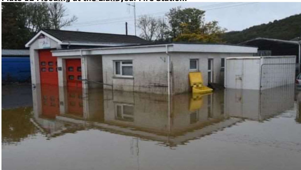
Plate 12 Flooding at the Llandysul Fire Station.
