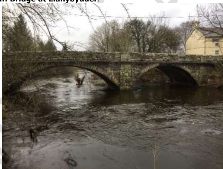
Plate 8 River Teifi Bridge at Llanybydder.
