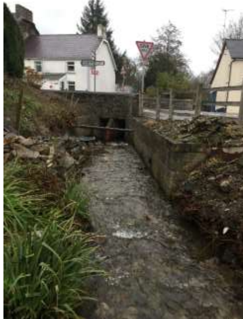
Plate 9 Photograph of the Nant Einon upstream of the B4337 highway culvert.
