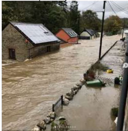
Plate 14 Flood water at Lewis Street, Pont Tyweli.
